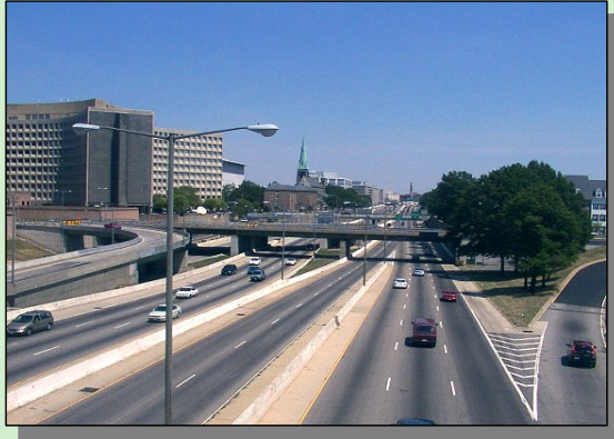
Colored pavement delineates the shoulder on this highway in the Washington, D.C. area
