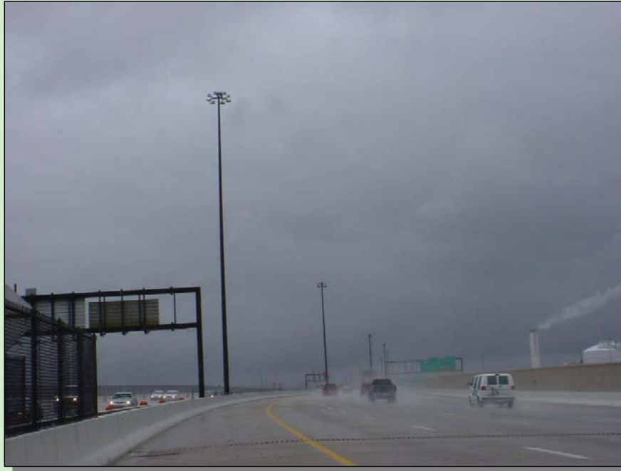
Light Fixtures along I-95, south of the Fort McHenry Tunnel
