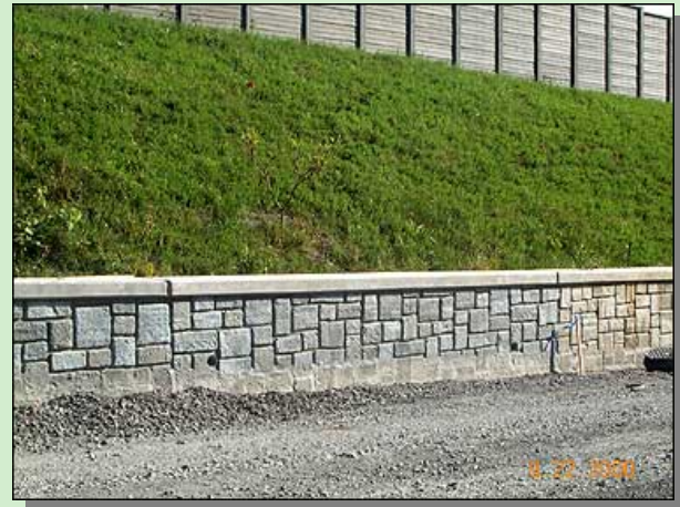
Retaining Wall with a Stone Pattern Concrete Formliner Finish
