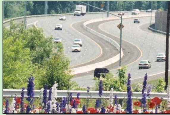
Colored Pavement Shoulders along I-495 in the Washington, D.C. area
