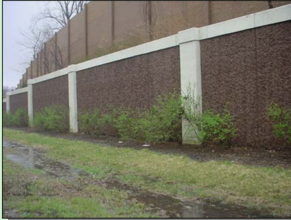
Retaining Wall with a Natural “Bark” Pattern Concrete Formliner Finish
