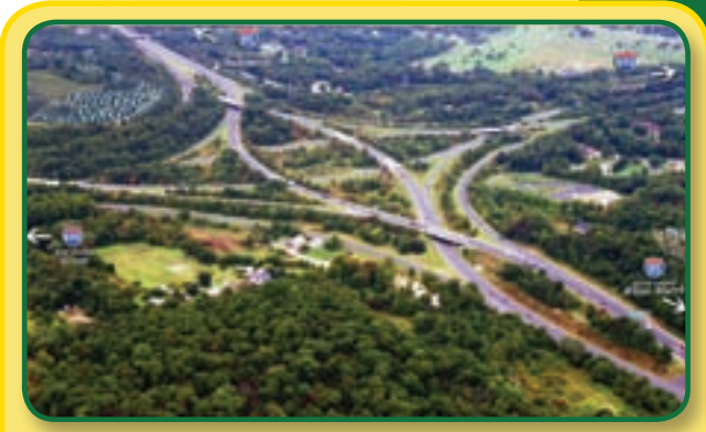
Above: I-95/I-695 prior to Phase I Construction
