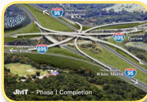
Above: I-95/I-695 Phase I Completion.
