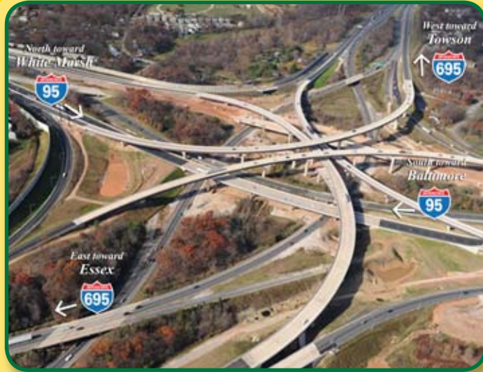
Above: The project area as of November 2009.
